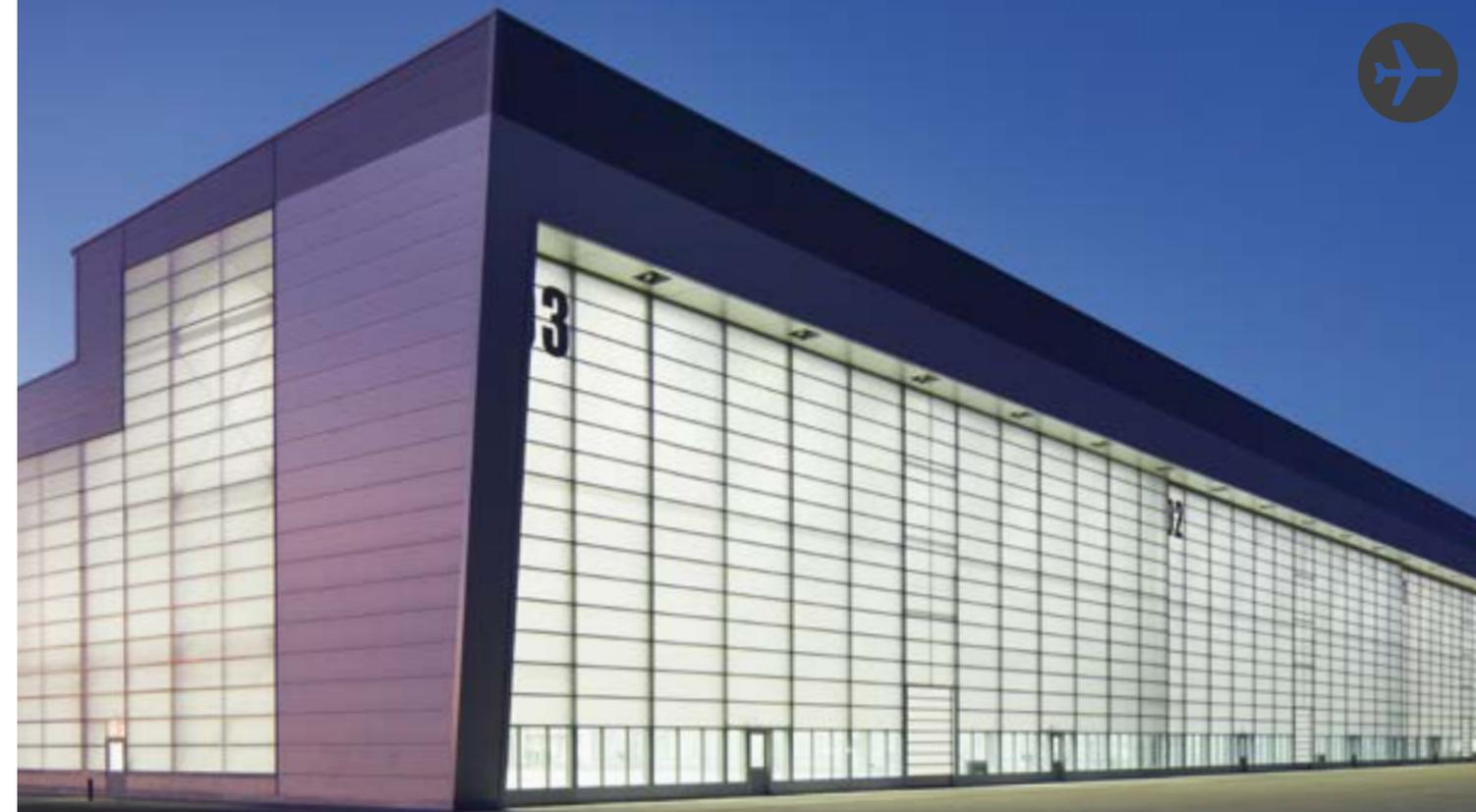
Door and façade elements made of translucent fibreglass create an interesting appearance, especially at night.
